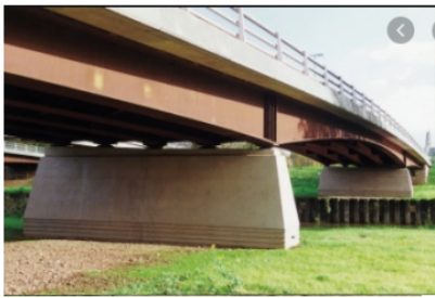
Example of Corten Weathering steel bridge beam
